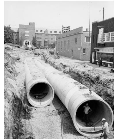
College Creek culverts being assembled, 1963
