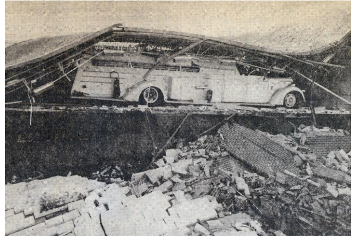
Fire Station after wall collapse, 1969 Photo credit Ames History Museum
